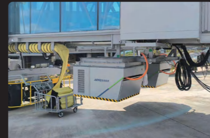
Lijiang International Airport
