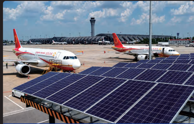
Chengdu Shuangliu International Airport
