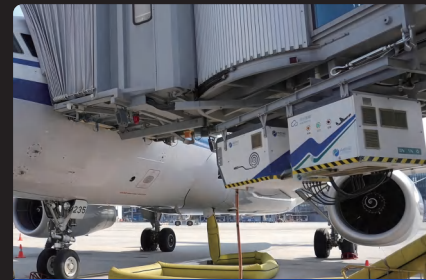
Hangzhou International Airport
