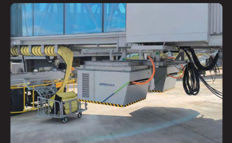
Lijiang International Airport
